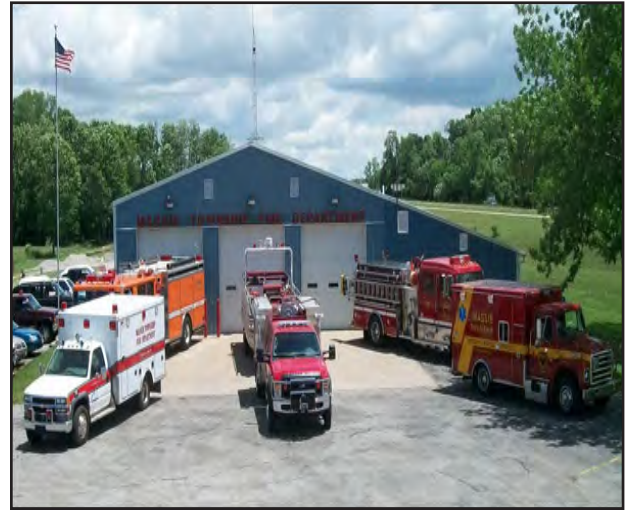
Figure 3.7: Massie Twp. Government Center & Fire/EMS Station
