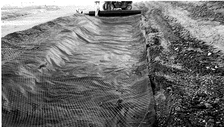
picture #2 Goetextile placed
