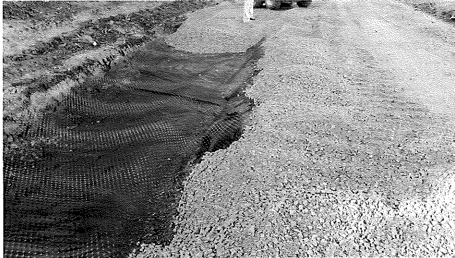
picture #1 Undercut #304 placement for compaction
